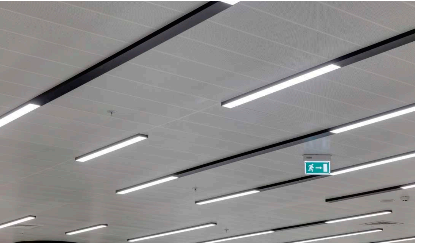
PROJE | SHEREMETYEVO ULUSLARARASI HAVALİMANI C TERMİNAL BİNASI / RUSYA PROJECT | SHEREMETYEVO INTERNATIONAL AIRPORT C TERMINAL BUILDING / RUSSIA İÇ MİMARİ | RMJM MİMARLIK INTERIOR DESIGN | RMJM ARCHITECTURE
